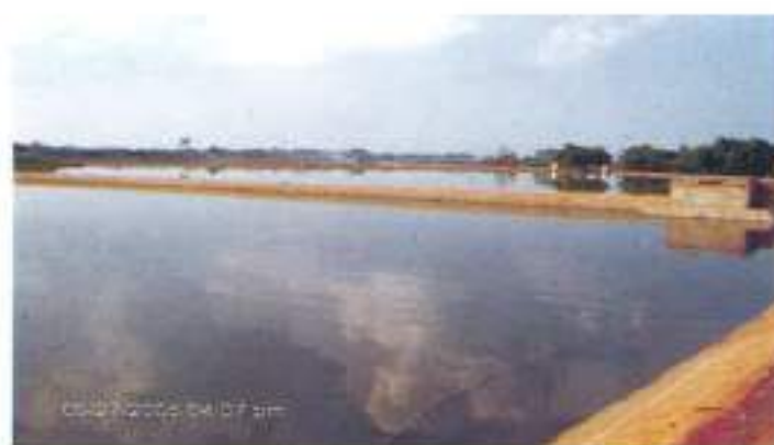
Plate 4.3 Sewage treatment through Oxidation Pond at Karuvadikuppam, Pondicherry
